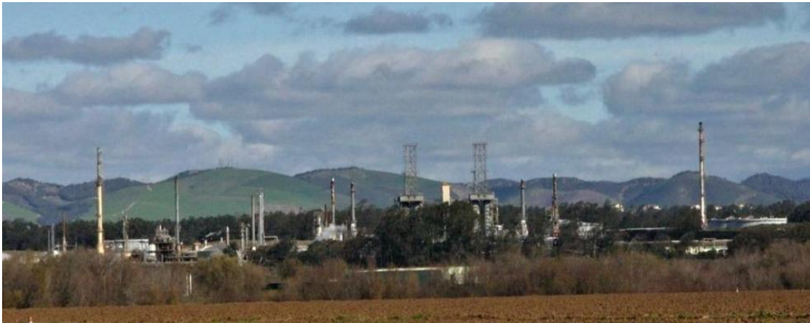
The now closed Phillips 66 refinery is now being cleared for its next use.
